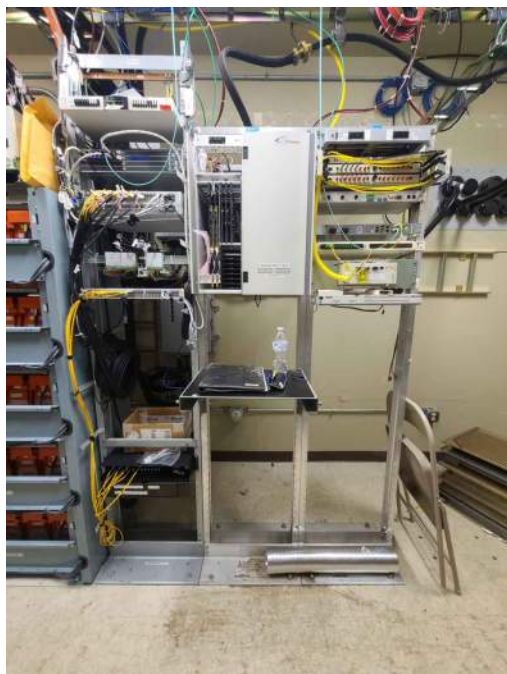
F EX. EQUIPMENT RACKS SCALE: NONE
